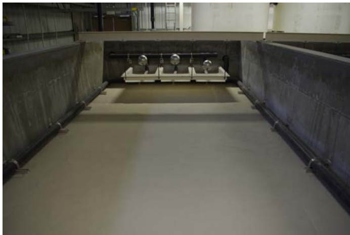
Figure 15. Filter cell before commissioning.
