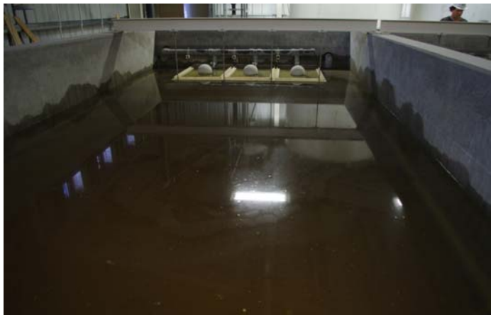
Figure 15. Filter cell before commissioning.
