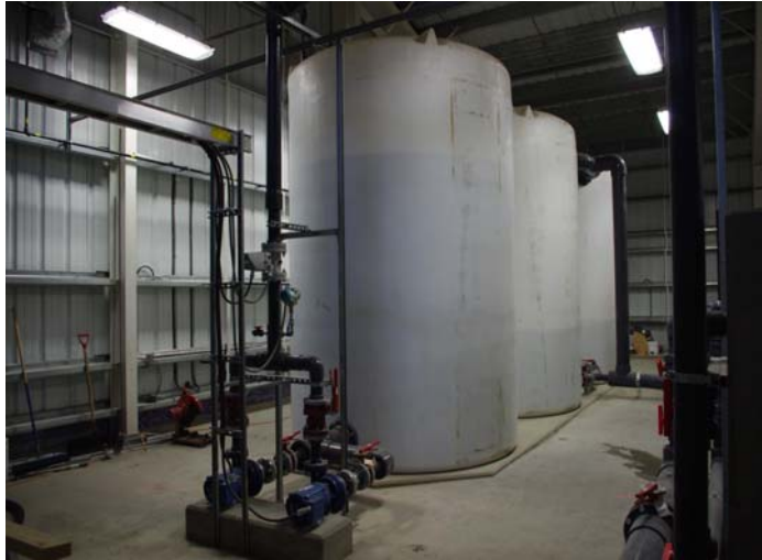
Figure 14. Contact tanks and transfer pumps.
