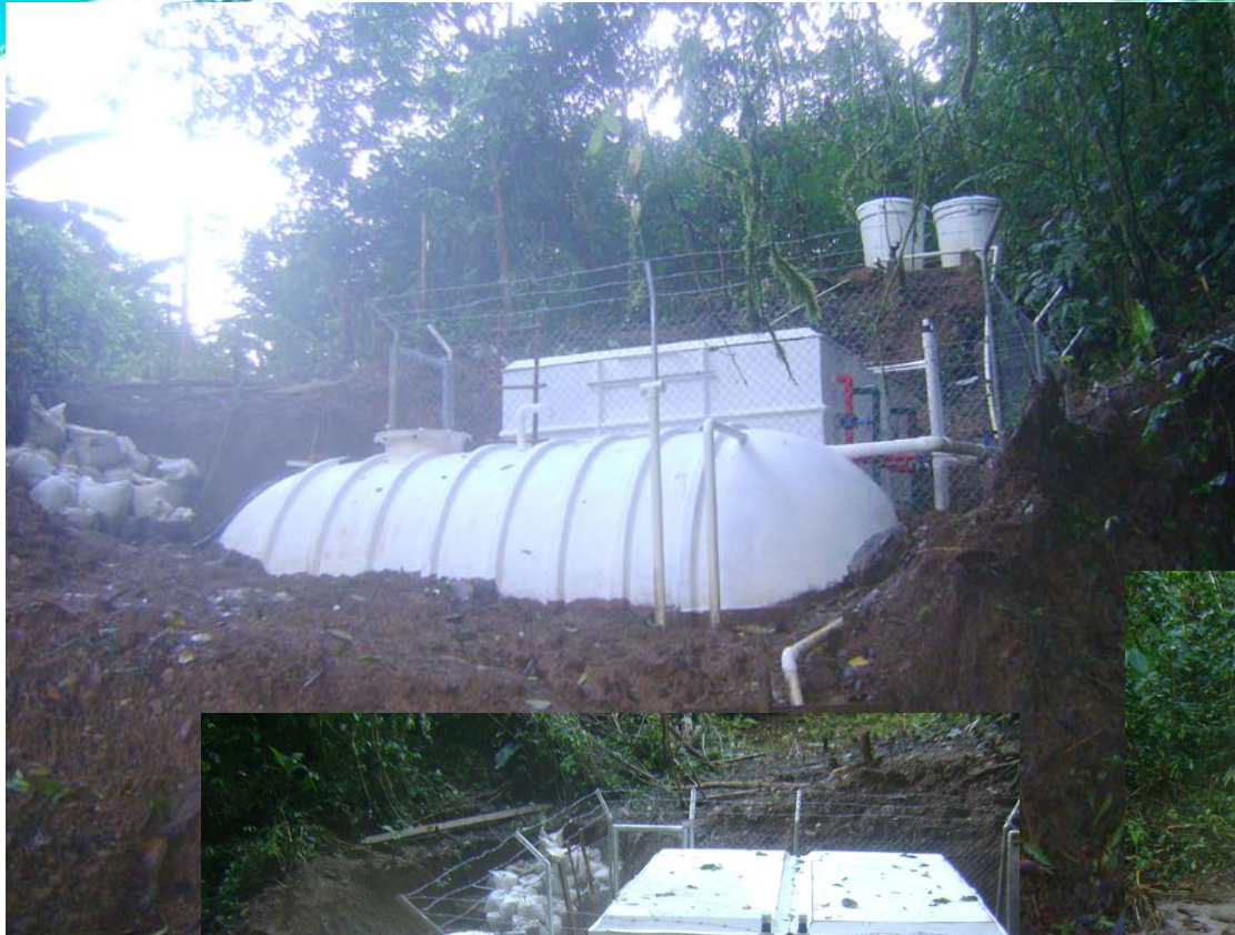
Fibre glass 4500 LPH MSSF Treatment System in Chocó, Colombia.
