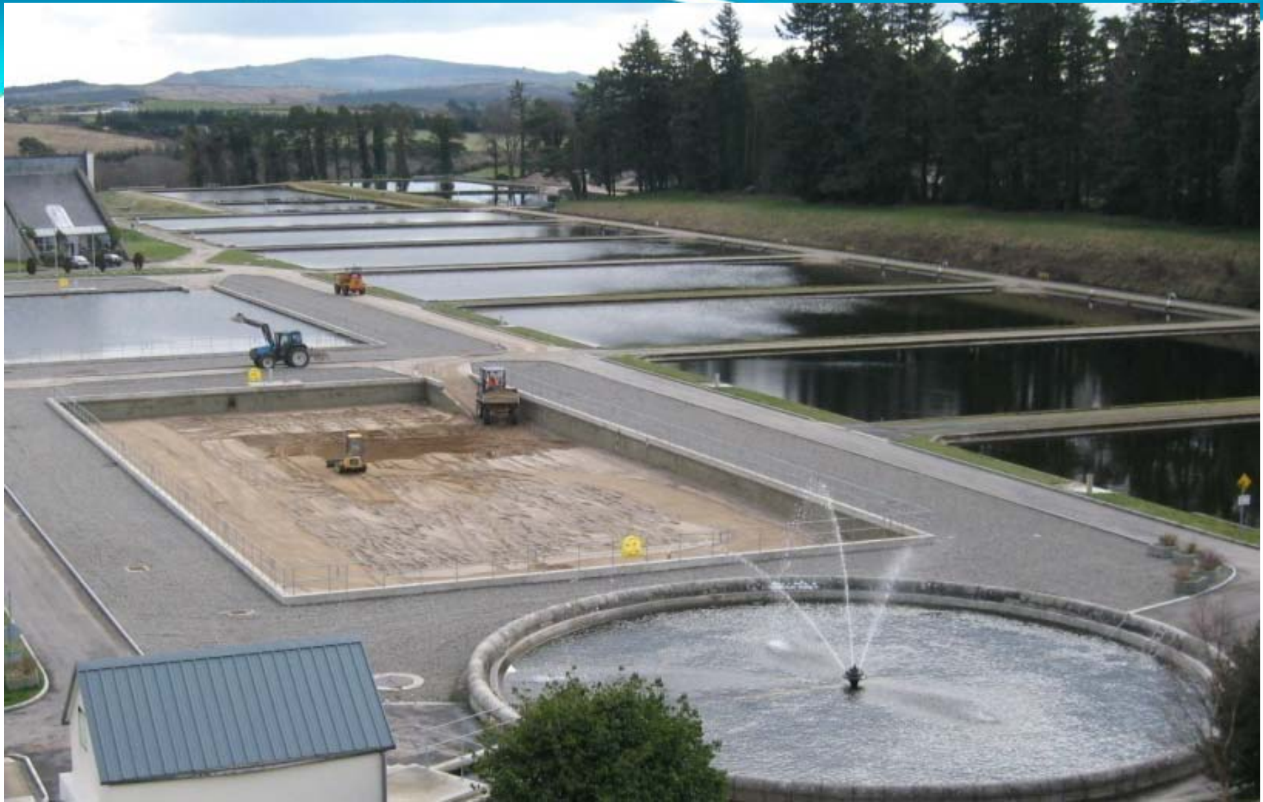
Cleaning a filter at the Vartry WTP near Dublin, Ireland
